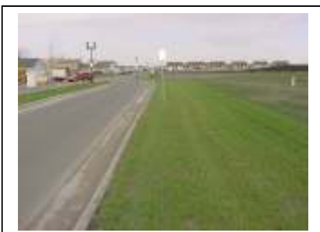
Filter strip protecting the curbline
