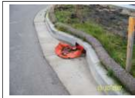
Street Inlet Protection
