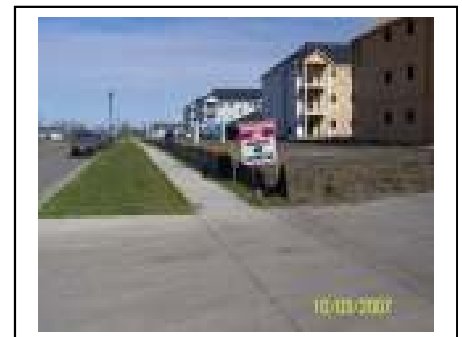
Filter strip used in addition to silt fence
