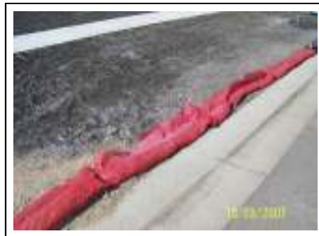
Rock wattles protecting curbline
