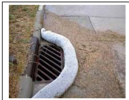
Pea gravel wattle around street inlet
