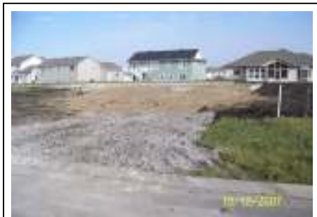
Rock entrance on a residential site
