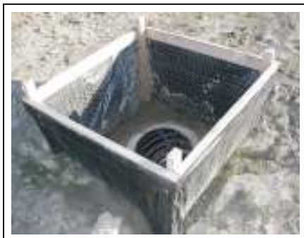
Constructed filter using silt fence
