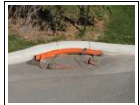
Street Inlet Protection
