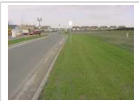
Filter strip protecting the curblin
