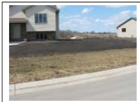
Filter strip used as a residential control
