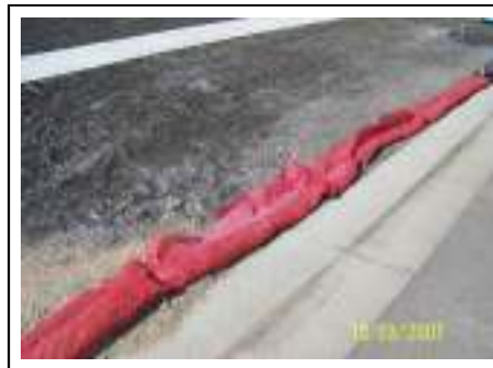
Rock wattles protecting curbline
