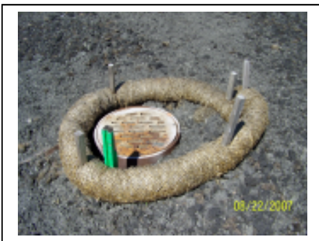
Straw wattle used to protect inlet
