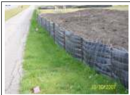
Silt fence with wire mesh backing
