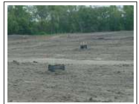
Constructed inlet protection
