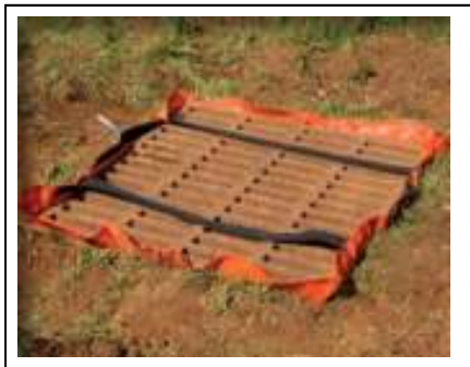
Drop down inlet protection device
